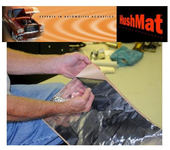
8. You simply peel the wax backing paper off of the HushMat Ultra sheets as shown here. The sheets adhere very nicely to the surface. A good idea is to think ahead of the process and trial fit the pieces before peeling the backing paper off and pressing into place.
