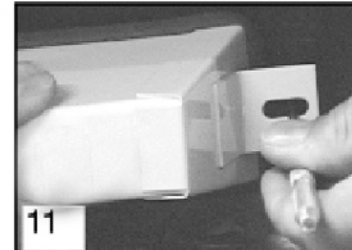
Position the light box and mark the position for the T-bolt studs.
