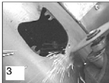
When you are satisfied with the position, scribe around the plate.
