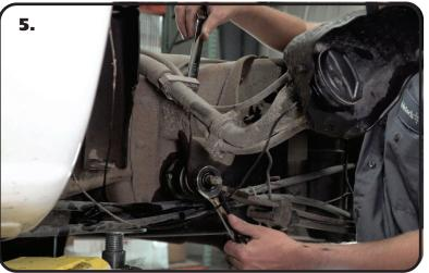
**5.** Loosen the front leaf spring bolts. You don't need to remove the nut and bolt.
