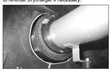
25. Fit the filter/drycharger assembly through the hole in the, onto the B-tube using the #44 hose clamp supplied. Ensure that the filter has sufficient clearance in the hole. If not, enlarge the hole as necessary.
