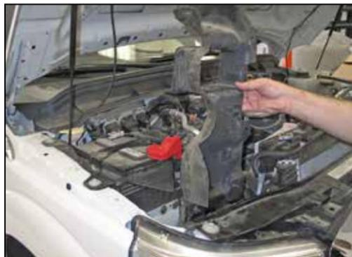
19. Remove the fresh air intake duct from the vehicle. Secure the inner fender to the vehicle with the original hardware from step #15.
