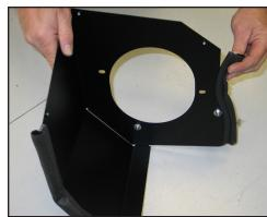
18. Install the remaining 11" edge trim onto the heat shield as shown.
