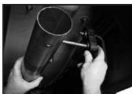
6. Insert hanger rod into isolator
