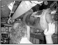
10. Remove factory muffler assembly.
