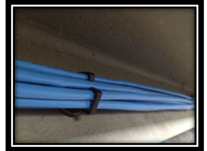
Picture above hiding 10 shielded Cat5e Cables inside an I-beam.
