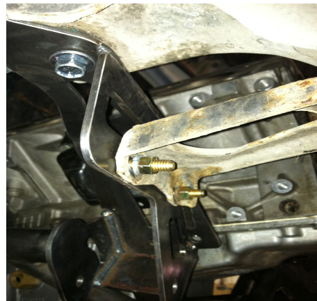
Fastening factory brace to UMI k-member
