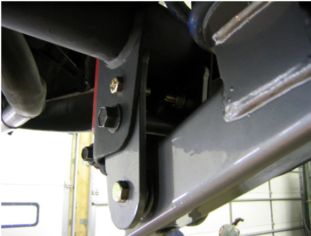
Image 4- Drivers Side Completed Installation, bolted not welded
