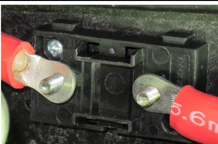
ALTERNATOR OUTPUT WIRE CONNECTED
