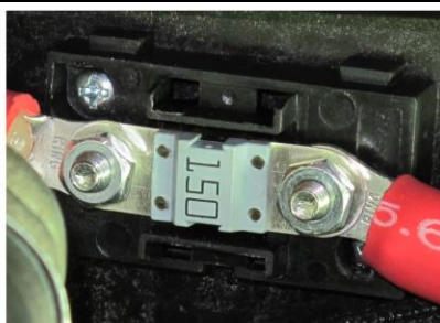
FUSE AND RETAINING NUTS INSTALLED
